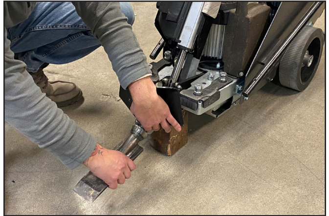
Installing the blade holder.
